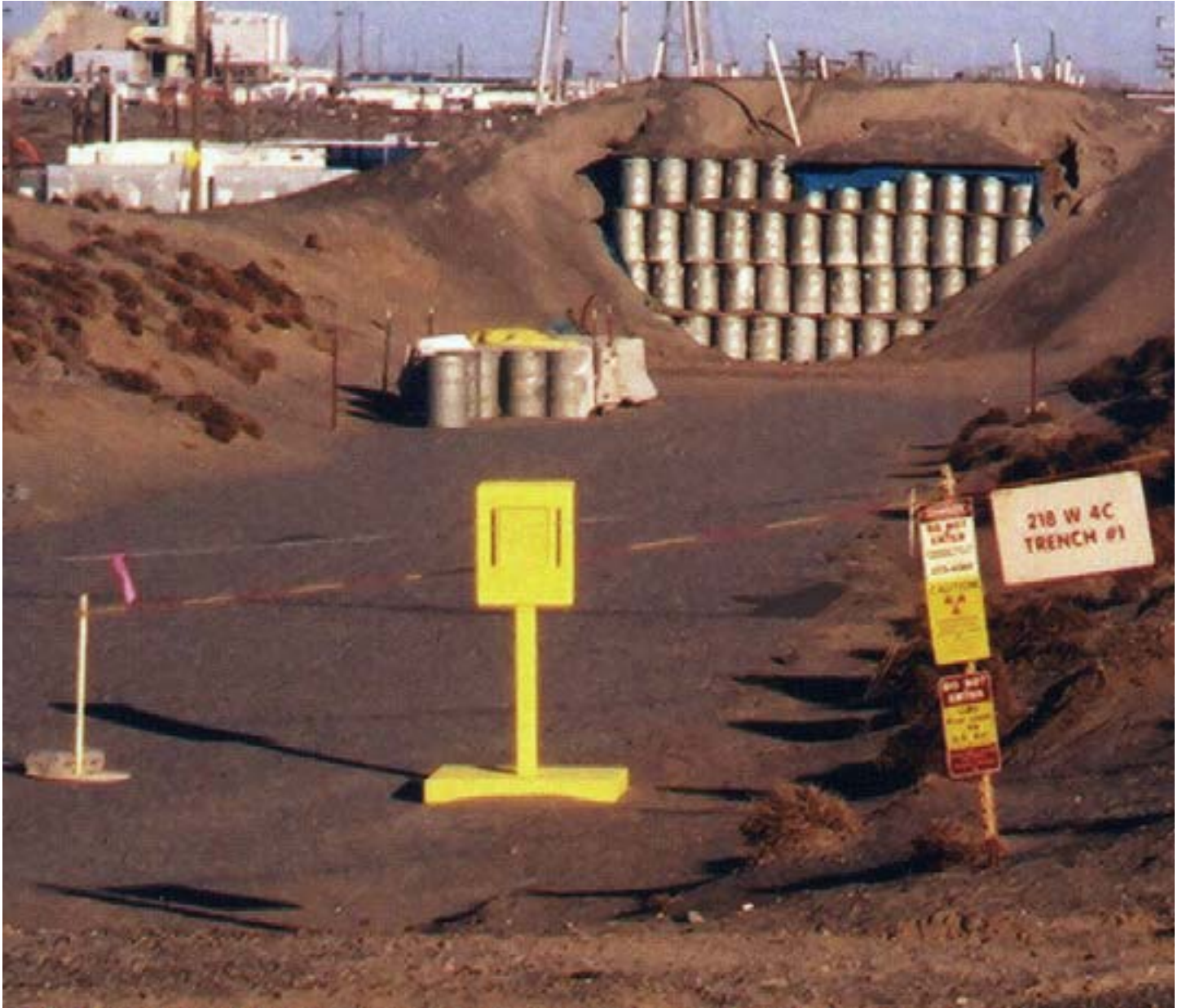
Burial Trench #1, an active unlined burial ground at Hanford. Barrels of waste are put into these burial trenches. There are no liners to separate the barrels from the surrounding soil.
